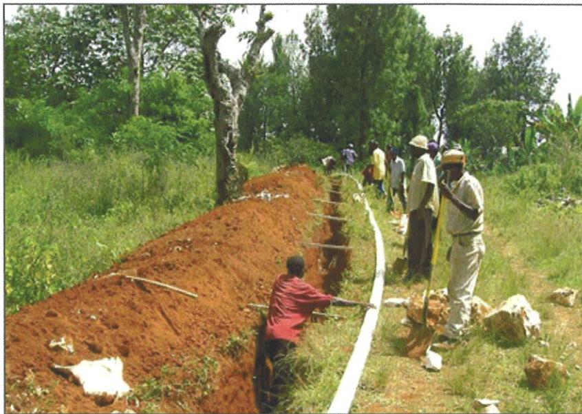
Workers excavate the trench by hand.
